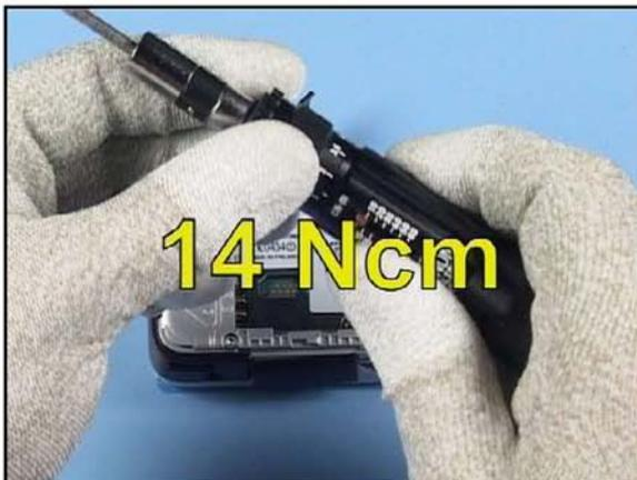
60. Set the torque driver to the correct torque.
